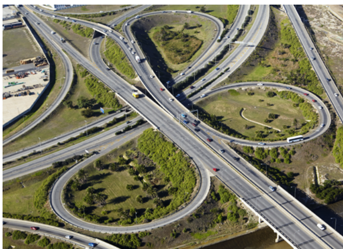
Legend: Aerial view of highway interchange – improved transport connectivity.
