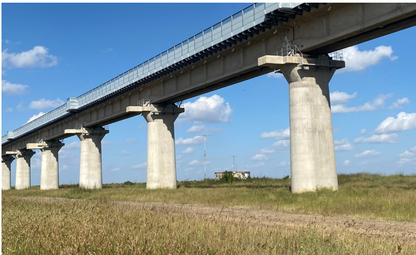
Legend: Elevated rail line through Nairobi National Park – modern rail infrastructure.
