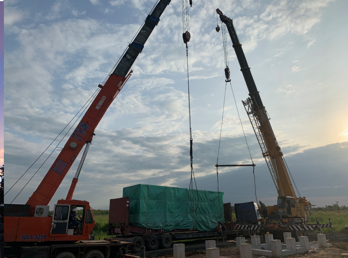
Box inverter lifting
