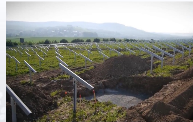
Profiled steel pile
