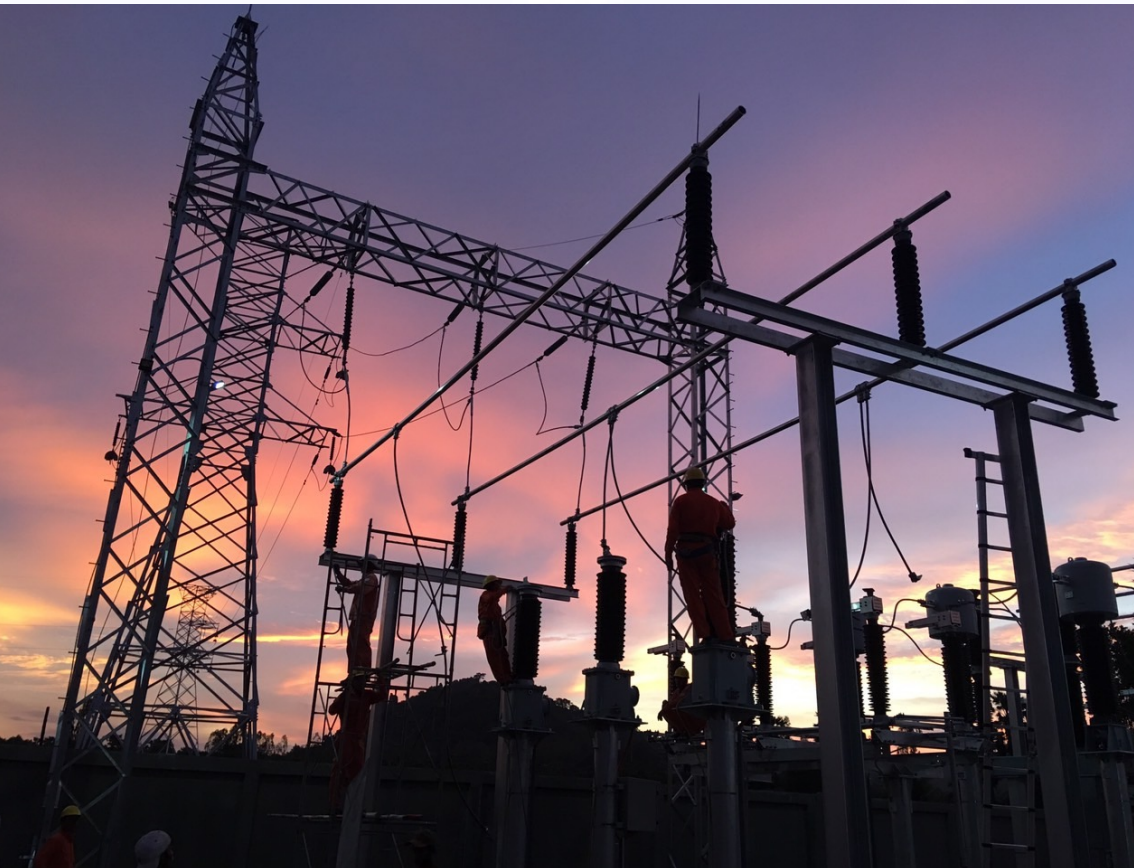
HV equipment installation
