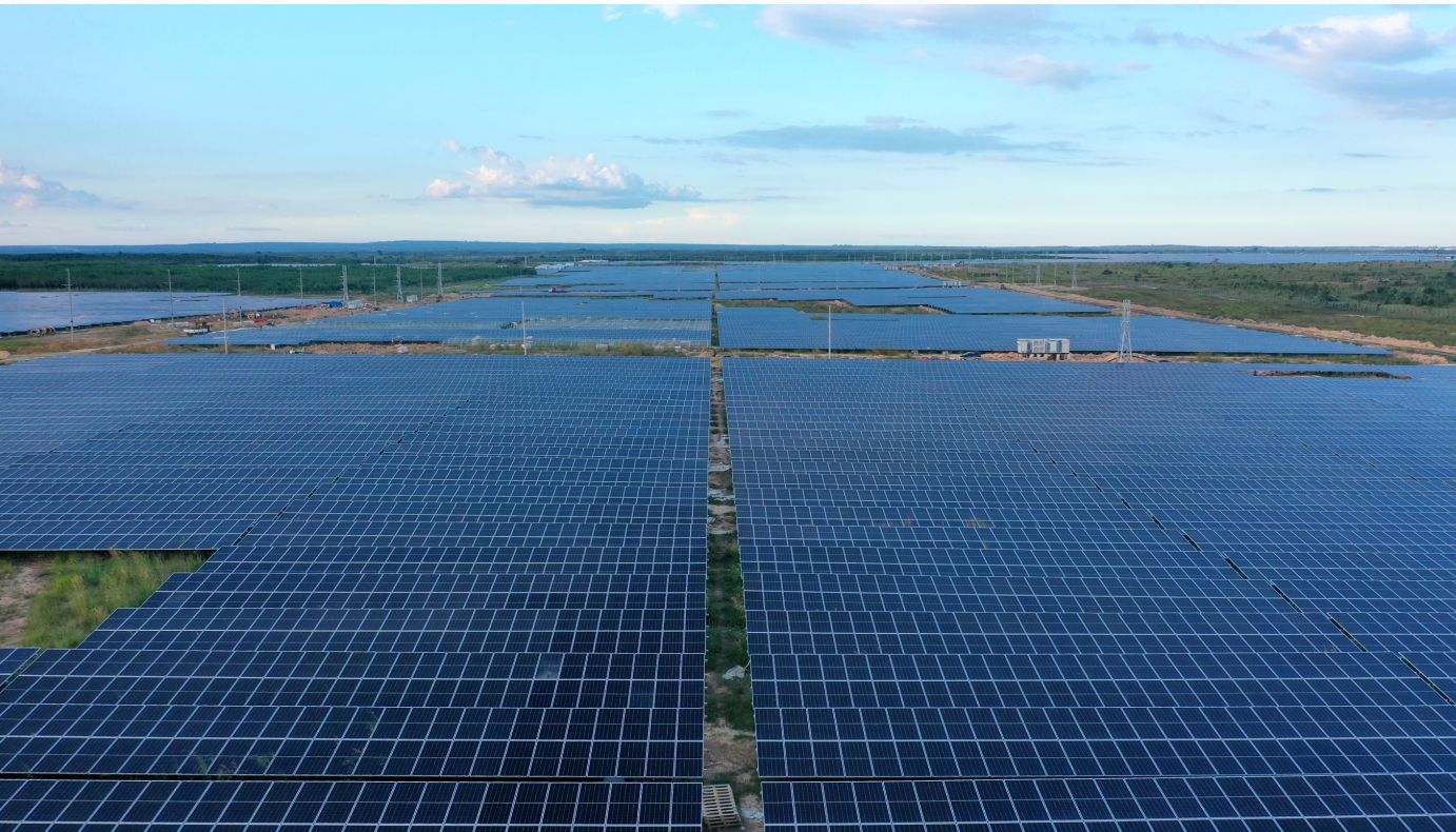
PV panel installation
