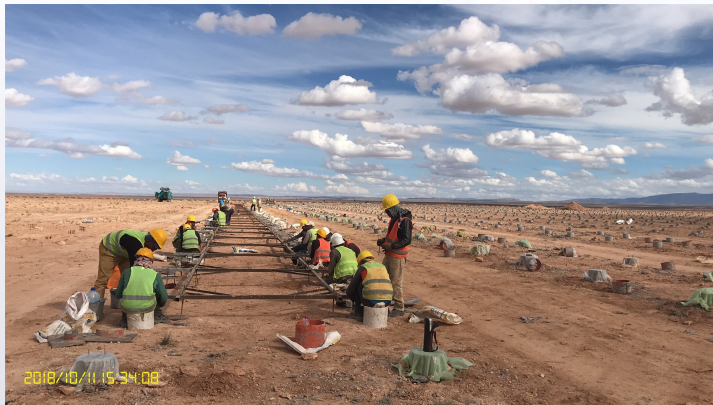
Cast-in-place pile
